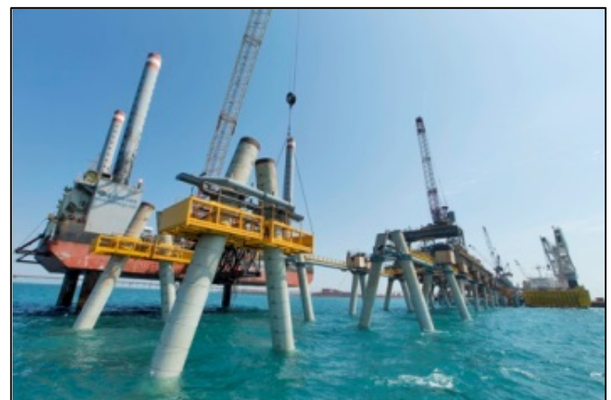
AEC Designed Workboxes, Friction Clamps and Wishbone Struts (copy of photo published in Engineers Australia Magazine, March 2013)
